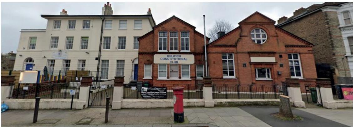
Figure 2: Existing building complex
