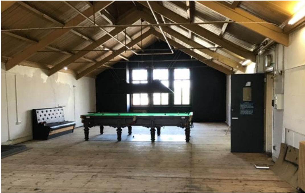
Figure 5: Central hall existing 1 st floor
